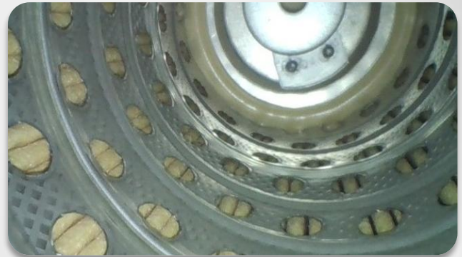
Lubrication Filter Inspection Using a 3.9mm VQ2 039 1500 4
