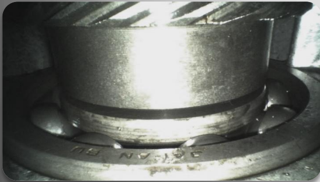
Gearbox Inspection Using a 6mm VQ2 060 1500 4
