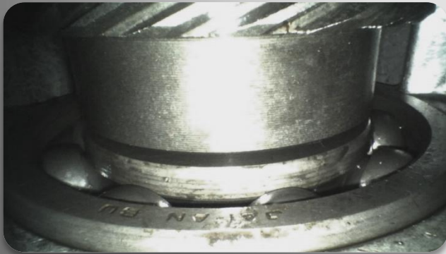
Gearbox Inspection Using a 6mm VQ2 060 1500 4
