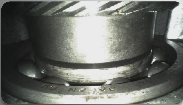
Gearbox Inspection Using a 6mm VQ2 060 1500 4
