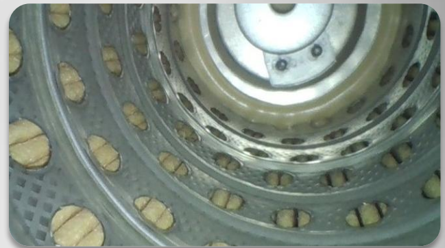
Lubrication Filter Inspection Using a 3.9mm VQ2 039 1500 4
